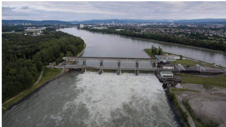
Weir Märkt at the hydro power plant Kembs (photo: Thomas Berwing; ©: https://creativecommons.org/licenses/by-sa/4.0/ ).
